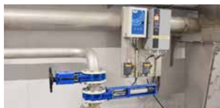
AVK knife gate valves with linear actuators on a reject water pipeline. The linear actuators were chosen, since they are energy efficient compared to actuators using compressed air
